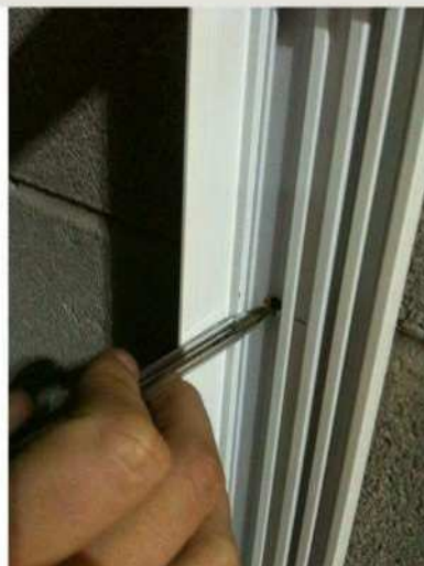
If rawl plug is required, mark position on wall through pre-drilled locations as shown.
