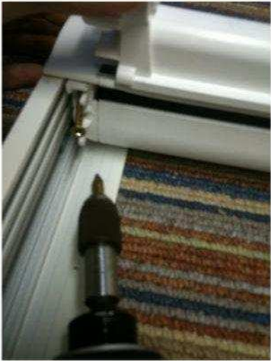
Fix cassette to block: Rotate handle and Insert screw provided into position
