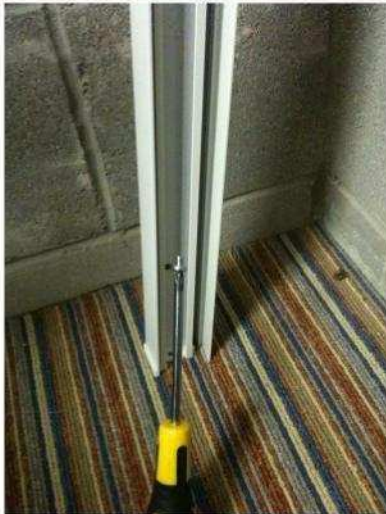
Take provided screws to be fitted through pre drilled holes in siderails
