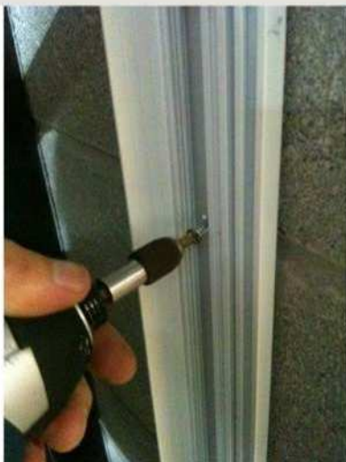
If no rawl plug is required, fix screw through pre drilled locations. Following Insertion of rawl plug screw in
