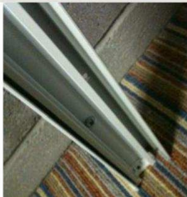
Slide siderail under cassette as shown and rotate the siderails into position
