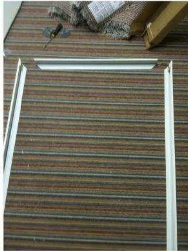
Begin by laying out three elements of recess mount frame as seen above.
