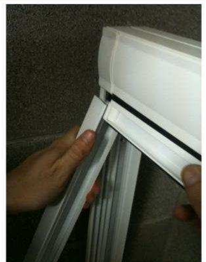
Fix siderail to cassette mount frame: Slide fabric into track of siderail as shown
