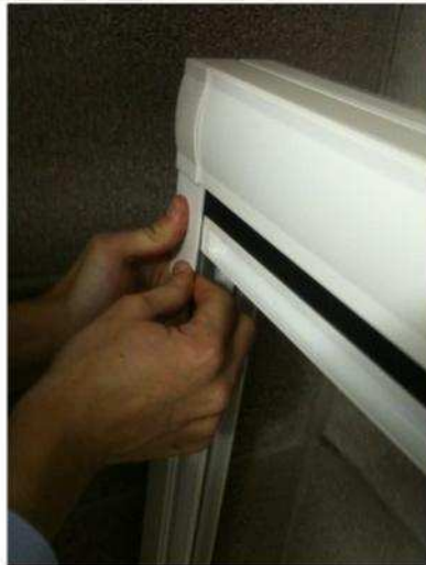
Slide siderail under cassette as shown and rotate the siderails into position
