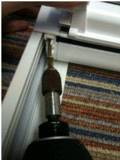
Fix screw into block. A cordless drill may be required to screw through into block. Repeat for right hand side
