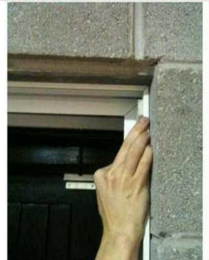
Raise assembled frame to mounting location. The frame is made to your exact specification.
